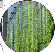
12 VINES AT MECHANICAL ENCLOSURE
